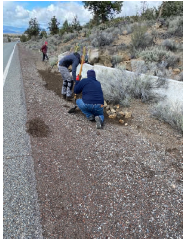
Ditch work Mar 24, 2024
